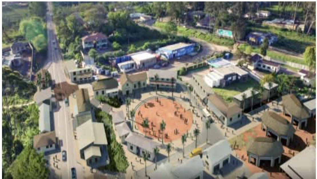
Umbumbulu Village, South Africa. Designed by Ubuntu Design Group in collaboration with the local Zulu tribal authority, municipal representatives, a nonprofit organisation, and the local community
